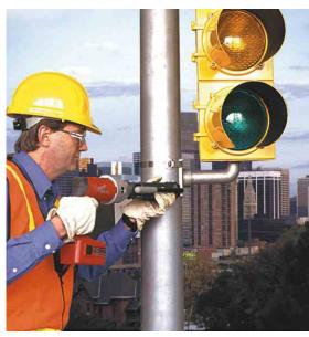
Traffic signals are quickly and easily applied with BAND-IT's Ultra-Lok clamps and a rechargeable, battery powered UL2000 tool.
